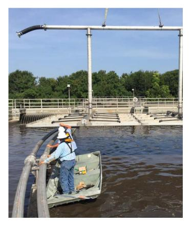
The Bosman<sup>®</sup> Plate Aerator<sup>imessilon</sup> has been retrofitted many different basins that previously used other types of aeration. Results of up to 50% energy savings have been achieved. Design and performance data is available for these retrofits.
