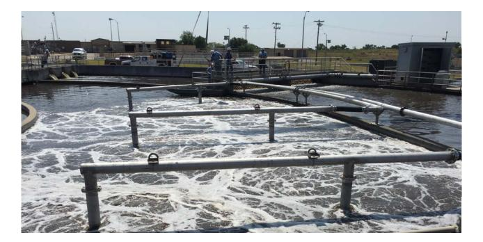
Since the Bosman<sup>®</sup> Plate Aerator<sup>™</sup> sits on the basin floor, volume and oxygen robbing grit and other detritus do not settle underneath and around it, as is common with nearly every other aeration system. This results in less basin downtime and maintenance.
